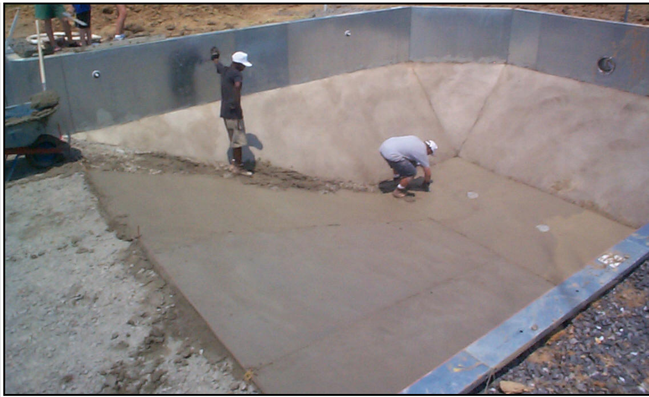
Pictures Showing Concrete Bottom Finish
