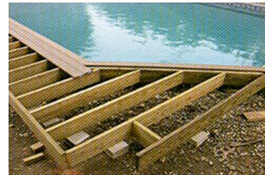
Wood Deck Framing
