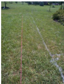
Pink String = Wall Placement White Paint = Over dig for 'Shelf'
