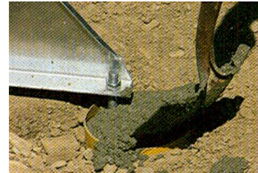
Concreting the Buttress
