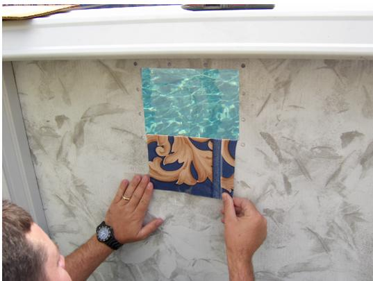
Pull down on flap and tape along the bottom edge.
