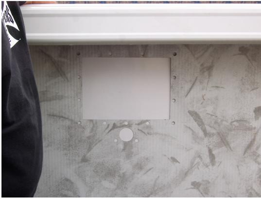
Once water level in pool has reached a minimum of 24 inches, the skimmer U gasket can be installed for skimmer installation.
