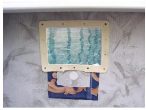
Install top half of U-gasket. Trim out a rectangle shape in liner as shown.
