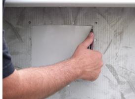
Start by using a flat piece of cardboard on opposite side to cut against. Trim by leaving a 1/4" strip between the knife blade and cutout edge. This allows the liner to stretch into position.
