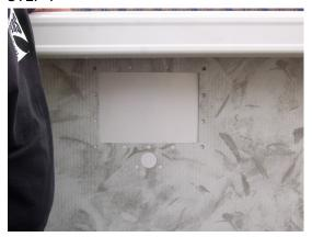
Once water level in pool has reached a minimum of 24 inches, the skimmer U gasket can be installed for skimmer installation.
