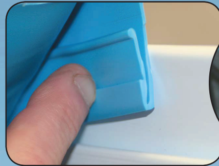
When your pool has a standard bead track, use the EZ Bead to slip right into the channel at the top of the pool wall. (Fig 2)
