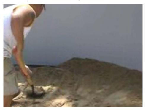
Once a 2" bed of sand has been made, a transition area for the liner to go from the pool wall to the floor must be made or installed. This transition area is called the cove. Cove can be made using an earth or using a pre-fabricated pool cove. The transition area should measure at least 6" up the wall and at least 6" out from the wall around the entire pool perimeter.
