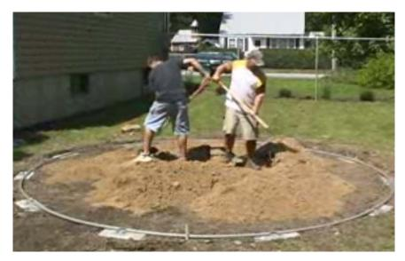
After all of the sand is brought into the center of the pool to be spread, replace the bottom track which was previously taken out.
