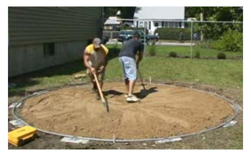
Spread out the sand to create a level area to place the wall while installing it into the bottom track. This layer of sand should not be under the patio blocks, bottom plates or bottom track.
