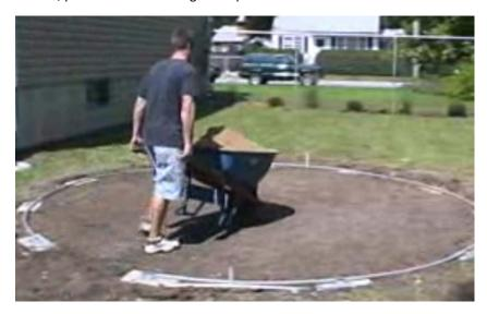
The bottom track of an above ground pool must rest on <u>solid ground</u>, not 'fill' or sand. Each of the bottom plates must have a patio block under them. The patio blocks should be recessed into the ground such that the top of the patio block is level with the ground and all blocks are within 3/4" of level to all the blocks. Once this is done, sand can be brought inside the pool bottom frame by removing one of the bottom tracks.
