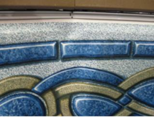
The weight of the vinyl pulling down will keep the bead in the coping. Make sure that the points around the perimeter of the liner floor match up with the panel joints of the pool wall. All wrinkles must be removed before filling with water.
