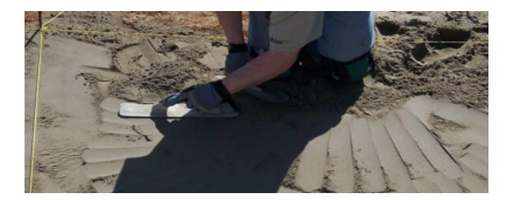
Spread the bottom material around the floor of the pool and **COMPACT** it to cover the string lines as you go. Use the edge of a flat board (about 36" long) to scrape the excess bottom material to expose the string lines. Run a trowel across the surface to smooth it out. A rounded bottom trowel works best. Remember to pull your pins and fill in their divots as you progress.
