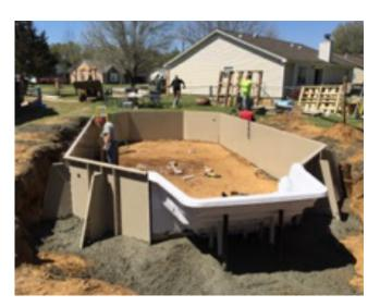
The concrete bond beam needs to be a minimum of 2500 PSI truck mix.
