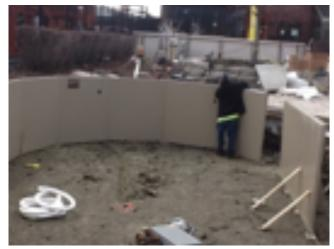
smooth liner installation and a flush top seat fit. Use a level to make sure that the pool walls are both plumb and level. Finish by driving the 18" rebar into the ground through the holes at the bottom flange on the back of panel. Make sure rebar is installed to correct depth. No more than 3" should be exposed when finished.
