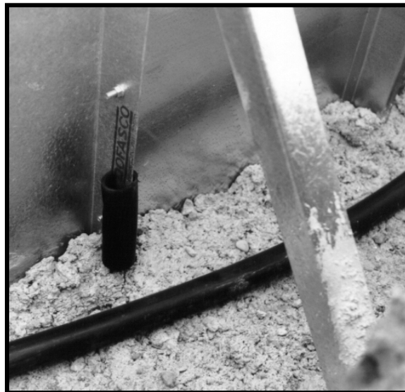
Run piping to bottom of excavation for support.
