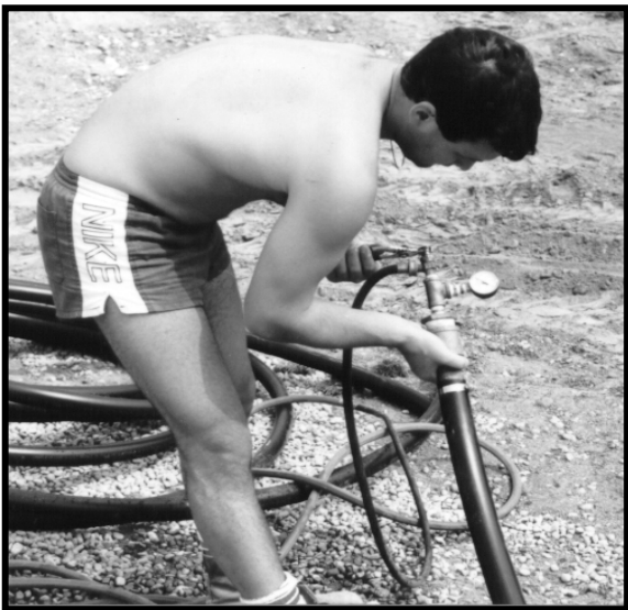
Pressure test all lines before backfilling.
