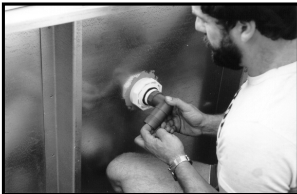
Thread the pipe adapters into the fittings.
