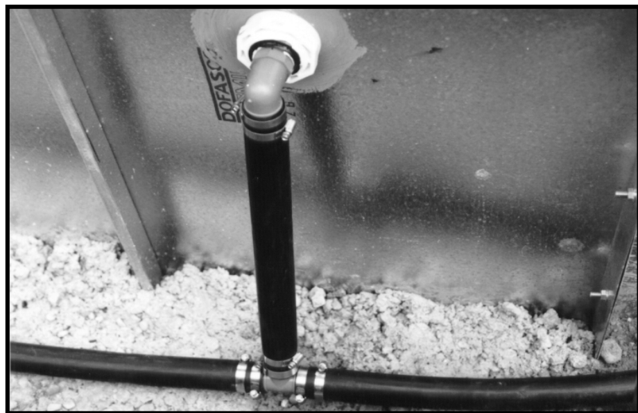
Run piping to bottom of excavation for support.
