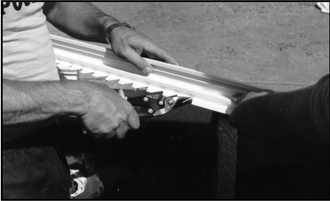
V notch coping for reverse curves.
