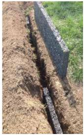
**HydroBlox HydroPlanks** are a permanent solution superior to traditional drainage. The product's high-void structure allows for a drainage capacity and structural stability greater than stone or pipe. Fast and easy to install, HydroPlanks redirect stormwater in any direction, without clogging. When installed, there is no need to connect the HydroPlanks, as the water moves from one plank to the next through the material. Simply install them so they are touching each other.
