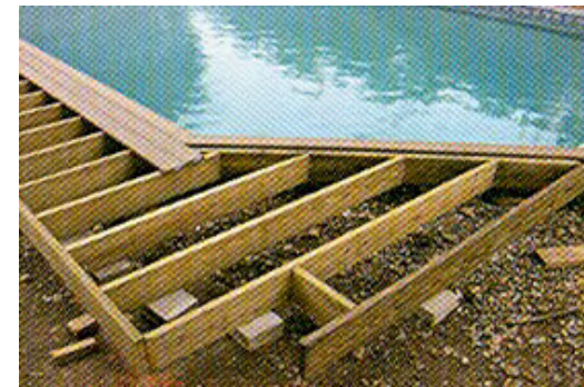
Wood Deck Framing
