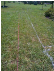
Pink String = Wall Placement White Paint = Over dig for 'Shelf'
