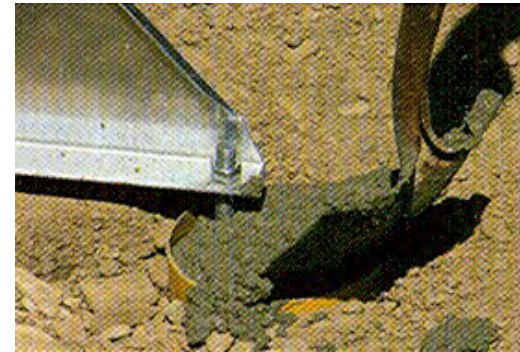
Concreting the Buttress
