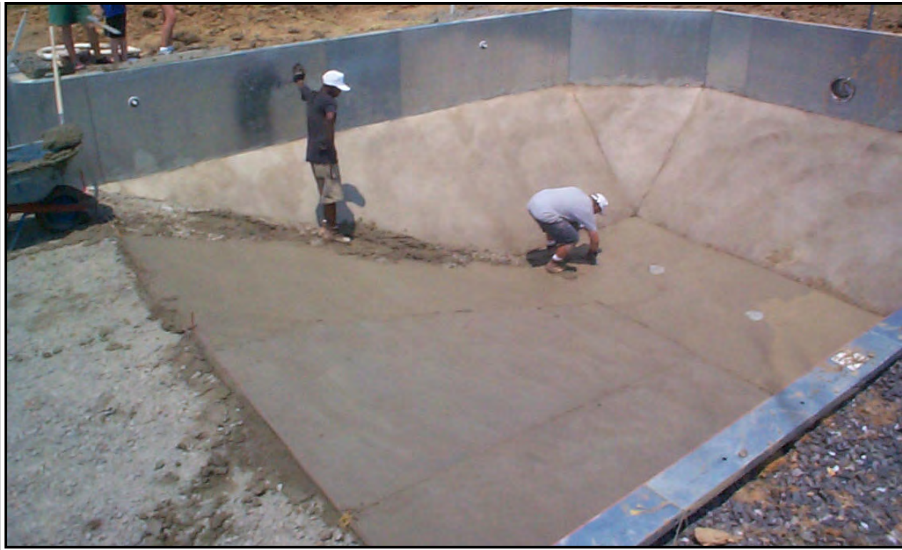
Pictures Showing Concrete Bottom Finish
