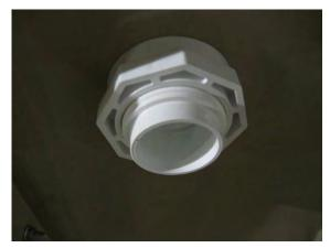
To install the return fitting, you need to un-thread the retaining nut from the fitting. Insert the threads through the prepunched hole from the inside of the pool and tighten the retaining nut to the back of the fitting. <u>Be careful not over</u> <u>tighten this nut.</u>
