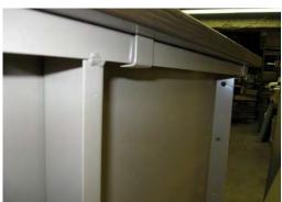
pool wall panel. The 90° angled bracket hooks under the outside of the panel top as shown in photo K.
