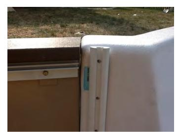
First locate the stair placement at the site. When using the "synthetic wood" top seat, the coping must be flush with the top of the cantilever stair as shown in photo B.
