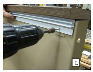
liner will not "pull down" the coping. These screw heads will be hidden after the liner is installed.
