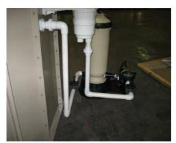
dealer for the proper sizing and filter media to meet your needs. When installing the plumbing lines, make sure that the skimmer is connected to the front (suction) of the pump and the return fitting is connected to the discharge side of the filter. Shut off valves are recommended for service and
