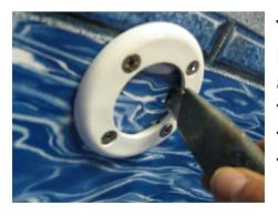
The return fitting face plate is installed in somewhat the manner as the skimmer. First find the round face plate and the pack of four faceplate screws supplied with the fitting. Note: there is <u>no</u> gasket installed between the liner and the return face plate. Press your finger against the liner to locate and mark the (4) holes. Screw down the faceplate with the #3 Phillips screw driver and cut out the center section of vinyl with the razor edge.
