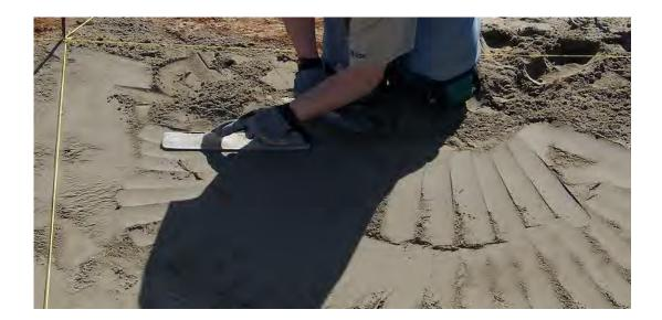
Spread the bottom material around the floor of the pool and **compact** it to just <u>cover</u> the string lines as you go. Use the edge of a flat board (about 36" long) to scrape the excess bottom material to expose the string lines. Run a trowel across the surface to smooth it out. A rounded bottom trowel works best. Remember to pull your pins and fill in their divots as you progress. "The last one out has to cover their tracks."
