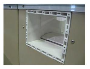
secure it using the two set screws supplied with the skimmer. If you have any questions, please refer to the manufactures installation instruction in the skimmer package.
