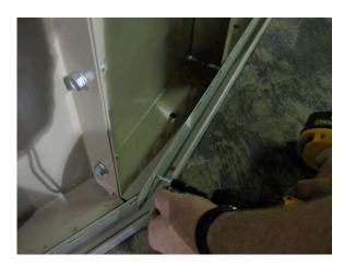
Install a section of "J" channel to the bottom of each panel following the same steps as the top installation.
