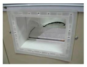
safety/warranty packet for later. Before installing the liner, double check the pool walls and the pool bottom for any dirt or sharp objects that could damage the vinyl material. Last but not least, make sure the skimmer and return gaskets are in place.
