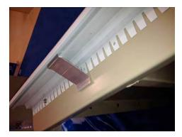
After the coping is mounted, place a support bracket, on the back side, in the middle of each panel and behind each coping joint. Lock the bracket into the back of the coping and fasten it to the top of the panel using one of the self drilling screws. Finish the installation by snapping a coping cap over each butt joint.
