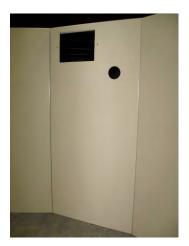
After all of the wall panels are placed around the site, it is time to begin the wall erection. Starting with the skimmer panel, align the front edge of the panel with the layout stakes in the location of your choice.
