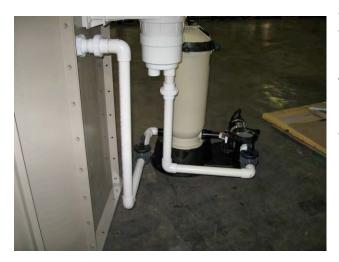
skimmer is connected to the front (suction) of the pump and the return fitting is connected to the discharge side of the filter. Shut off valves are recommended for service and maintenance on this equipment.
