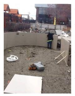
Secure the panels by using the 9/16" Galvanized nuts and bolts that were supplied with this package. Begin bolting the panels together using only the top two and the bottom bolt on each seam, until you have closed the circle. NOTE: Keep the panel connection on the outside of the layout stakes. We suggest that you <u>hand</u> tighten the panel bolts until the entire pool wall is erected.
