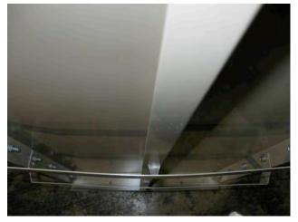
adhesive rubber bumper between the plate and the center wall stiffener as shown. The final phase is to install the vinyl siding. The vinyl siding is pre-cut to fit between the "J" channels we installed earlier on the top and bottom of the panels.
