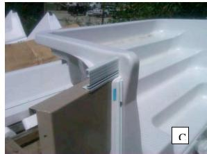
finished elevation is established, drill through the stair flange at each panel hole location using a 1/2" drill bit and bolt the panel to the stair.
