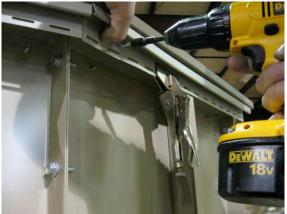
wall flange as shown. Each section of "J" channel is held on by four (4) of the self drilling self tapping hex read screws. Note: The slotted holes in the "J" channel are not used for this application.
