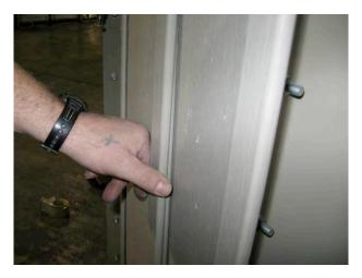
side of the skimmer panel. Secure the end pieces of siding to the stability plates using a hex headed self drilling self taping screw at each plate. This procedure will help prevent wind damage to the siding.
